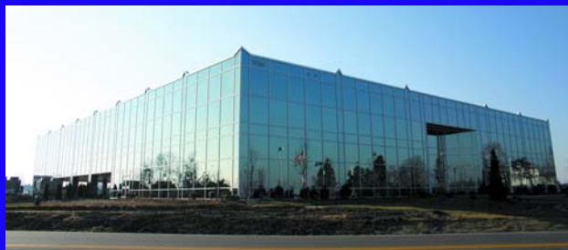
Southern Star Central Gas Pipeline 4700 Highway 56, Owensboro, KY
